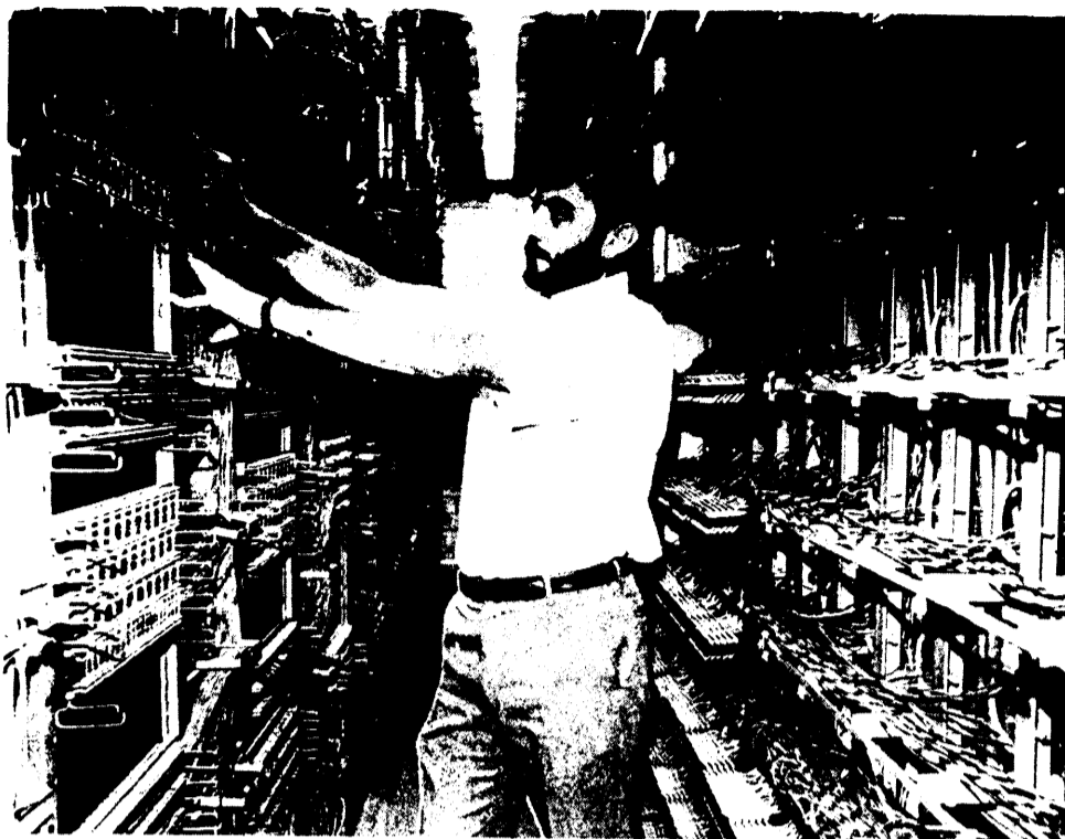
COMMUNICATIONS CENTER — Dennis Sugar, network supervisor for United Telephone Co., checks out some of the equipment in the company's switching office on Adams Street in Newton. (Pat Decker photo)
